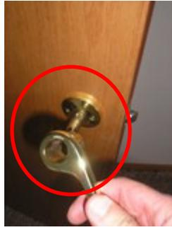
The lower level SE bedroom entry door latch needs adjusting to catch. The lower level NE bedroom door knob needs its setscrew tightened. The lower level sliding window tracks need to be cleaned to allow the windows to slide open and closed easily. The upper level north bedroom inner wooden window ledge is in need of surface preservative maintenance.
