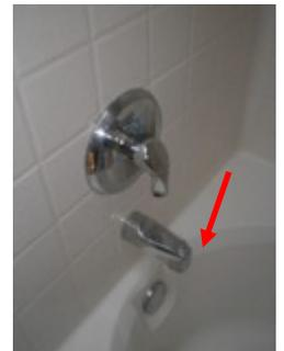
The master bathroom bathtub/shower faucet drips for an extended period of time after the valve is turned off. The other bathtub faucets stop dripping rather quickly, but this faucet does not. The seal is leaking in the upper level main bathroom toilet flush mechanism. This flush mechanism needs to be changed before water starts spraying up against the tank cover and water starts dripping behind the toilet.
